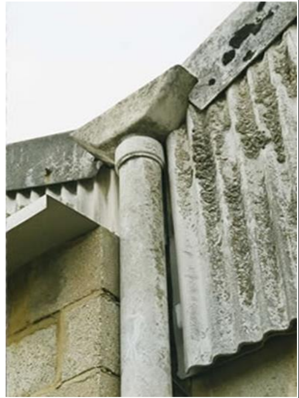
Asbestos cement downpipe, hopper and profile sheet
